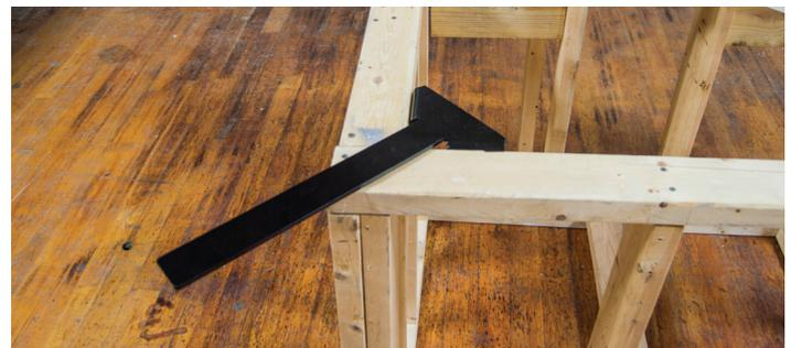
ers using a drill bit that is slightly smaller than the ¼" holes on the plate. When all the pilot holes are drilled, install your brackets in line with the Anthem Hidden Bracket. Be sure to check level beginning with your first bracket placement and then from bracket to bracket as you install.
